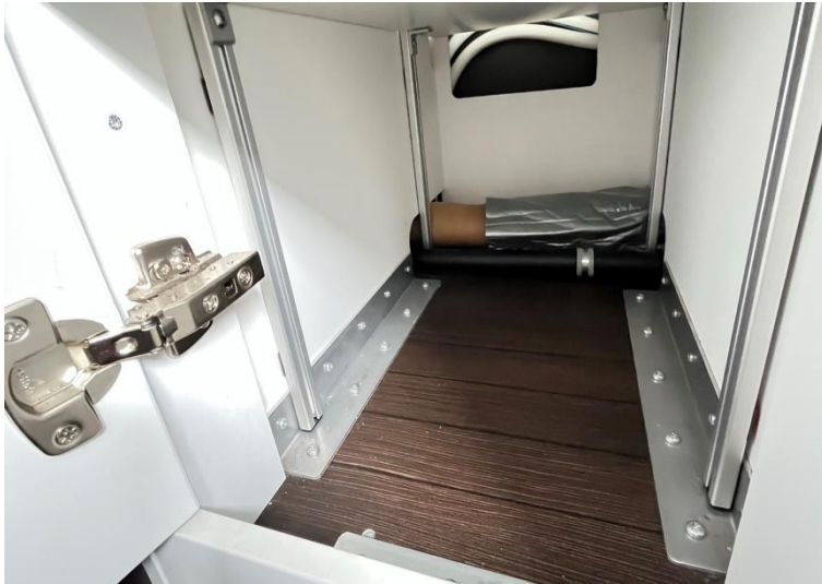
Figure 5. Positioning of aluminium tracks
